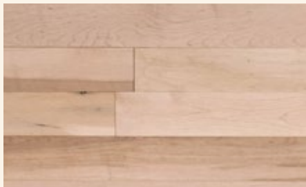
Joints too close together
